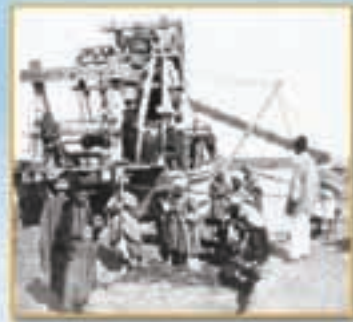
▲ Construction of the Suez Canal began in 1859 and took workers 10 years to complete. Although digging was first done by hand, laborers later used dredgers and steam shovels to remove sediment.
